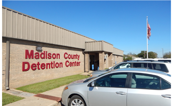
Madison County Detention Center
