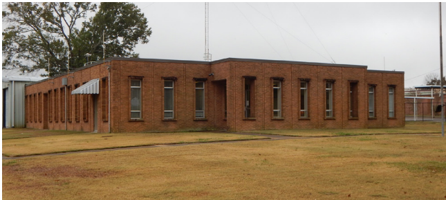
Madison County Emergency Services Complex
