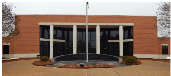
Circuit Court Building
