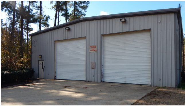
Southwest Fire Department, Station #1
