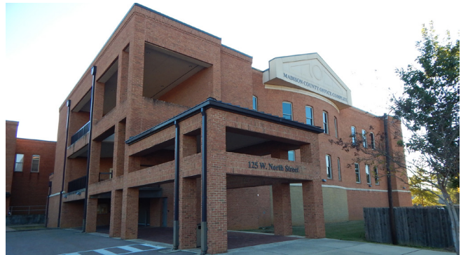
Madison County Office Complex
