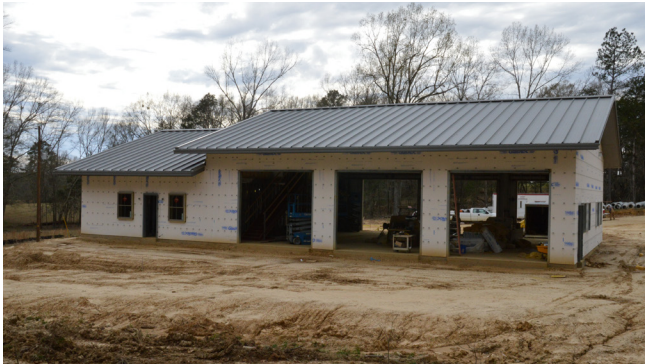
Southwest Fire Department, Station #2
