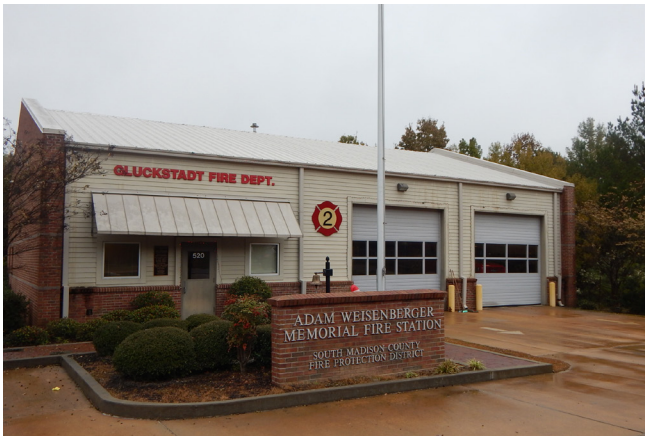
Gluckstadt Fire Department – Station #2, Stribling Road
